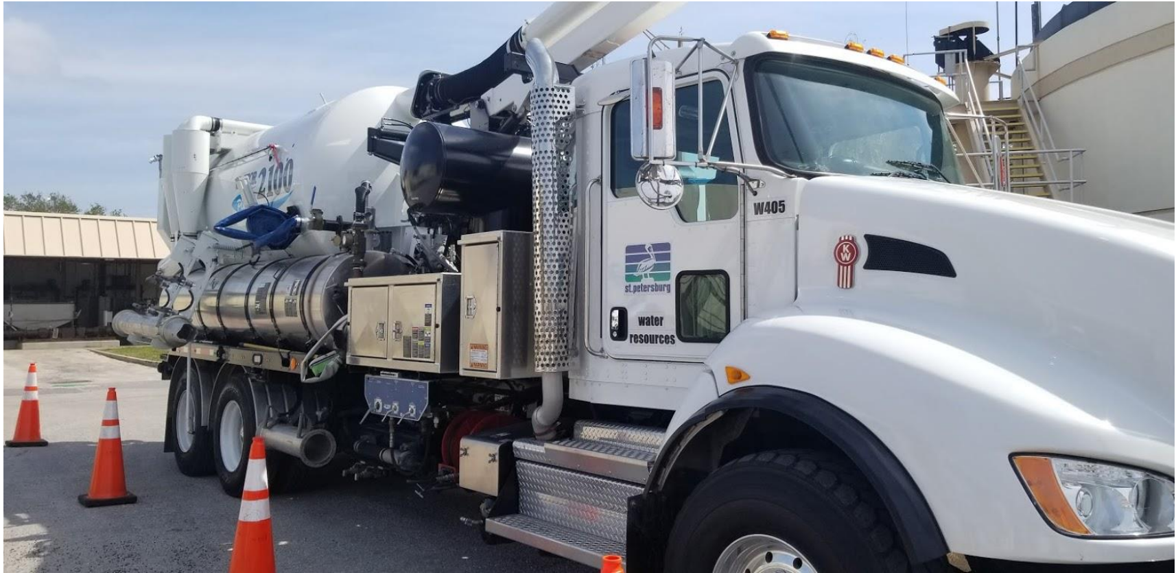
Snorkel truck for cleaning out blockages from the sewer.
